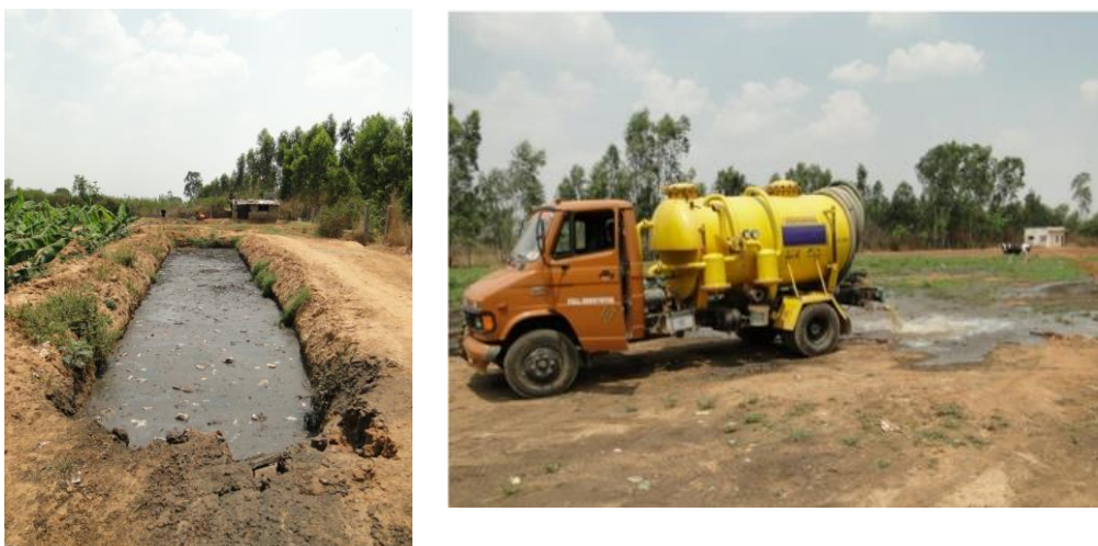
Figure 20: Storage and dewatering in a pit and on uncultivated land. Photo: V. Srikantaiah.
