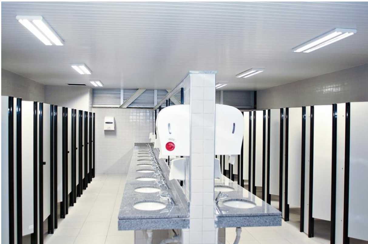
Figure 47: Vacuum toilets at UNINOVE University, Sao Paolo, Brazil 65 .
