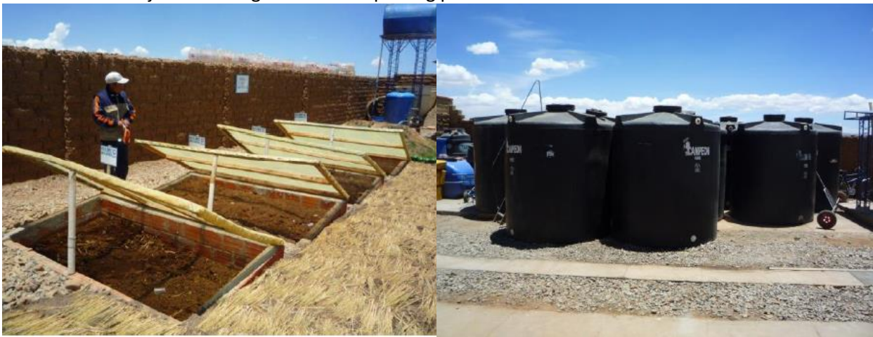
Figure 7: Composting trenches and urine storage at the compost center. Photos: K. Andersson.
