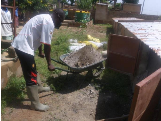
Figure 14: Emptying of a double-vault toilet. Note the dryness of the feces. Photo: L. Dagerskog.
