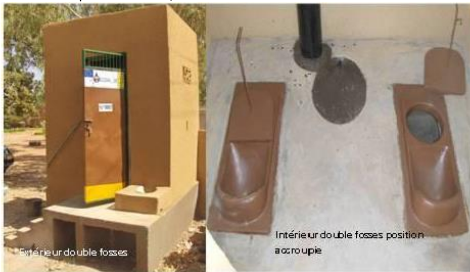
Figure 12: Double-vault, urine diverting toilet with squatting pan in Ouagadougou. Photos: CREPA.
