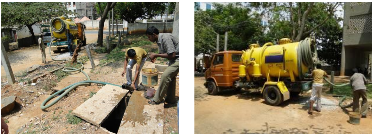
Figure 19: A private operator emptying a soak pit from a hostel building. Photo: V. Srikantaiah.
