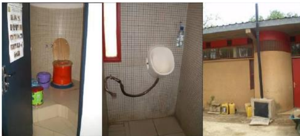
Figure 13: Urine-diverting toilet with urinal inside a house. To the right yellow jerry cans used for urine collection can be seen as well as the entry into the feces vault. Photo: A. Fall.
