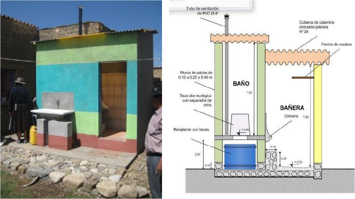
Figure 5: The toilet with shower and hand-washing basin from the exterior (photo: K. Andersson) and a drawing of the toilet with shower (source: C. Suntura).
